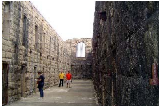
Inside the gaol
